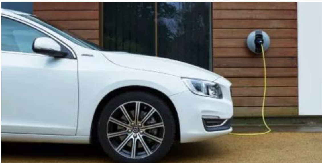
Figure 8. Residential charging point
